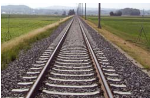
View of the noise measurement point with microphones on the left and on the right side of the track
